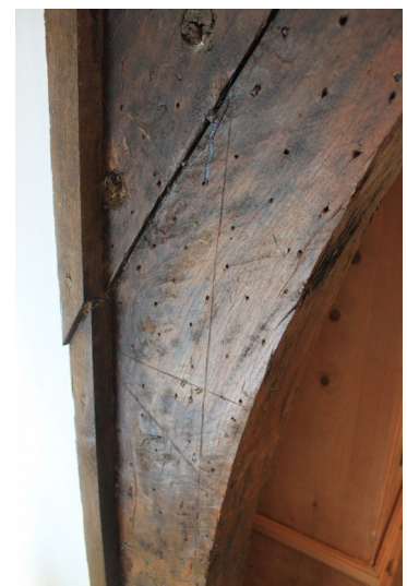
Jointed Cruck scratched layout marks.
