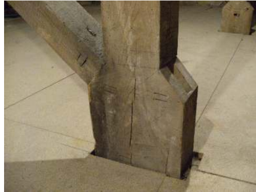
Fig. 23 Stogursey, High Street, No. 2, carpenters' marks (photo John Rickard)
