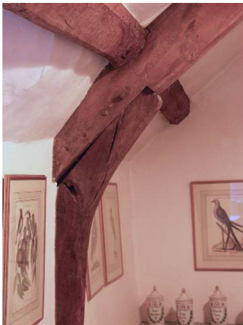
Fig. 7 High Ham, Hillbourne, jointed cruck (photo John Rickard)
