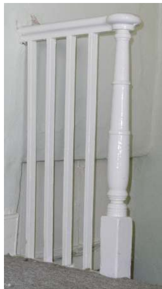
Fig. 24 Stogursey, High Street, No. 15, stair newel and balusters (photo John Rickard)
