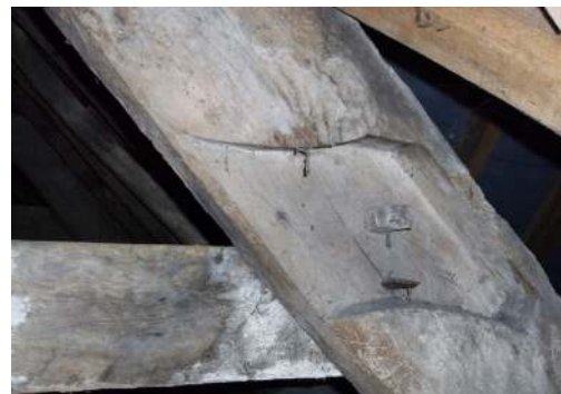
Fig. 18 Stogursey, Castle Street, No. 8, reused roof timber (photo John Rickard)
