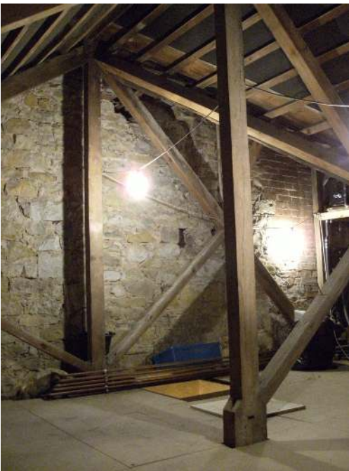
Fig. 22 Stogursey, High Street, No. 2, king-post truss (photo John Rickard)
