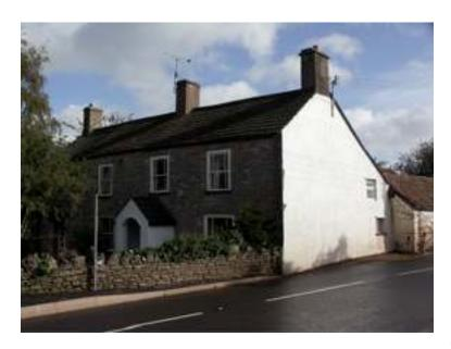
Originally, the house was a two-unit gable entry plan, one room being an unheated service room, dating from the 16th century. The house had an upper floor from the outset and would then have been one-and-a-half storey. In the early/mid-17th century the
