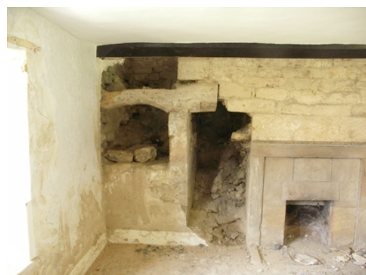
Fig. 7 Old Harp House, Over -Stratton, remains of bressumer and access to curing chamber
